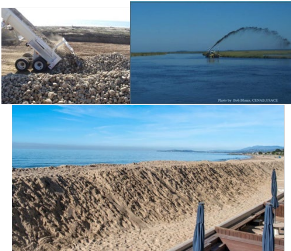
Figure 7. Images of cobbles (top left), fine sediment (top right), and sand (bottom) being utilized for enhancing coastal resilience.
