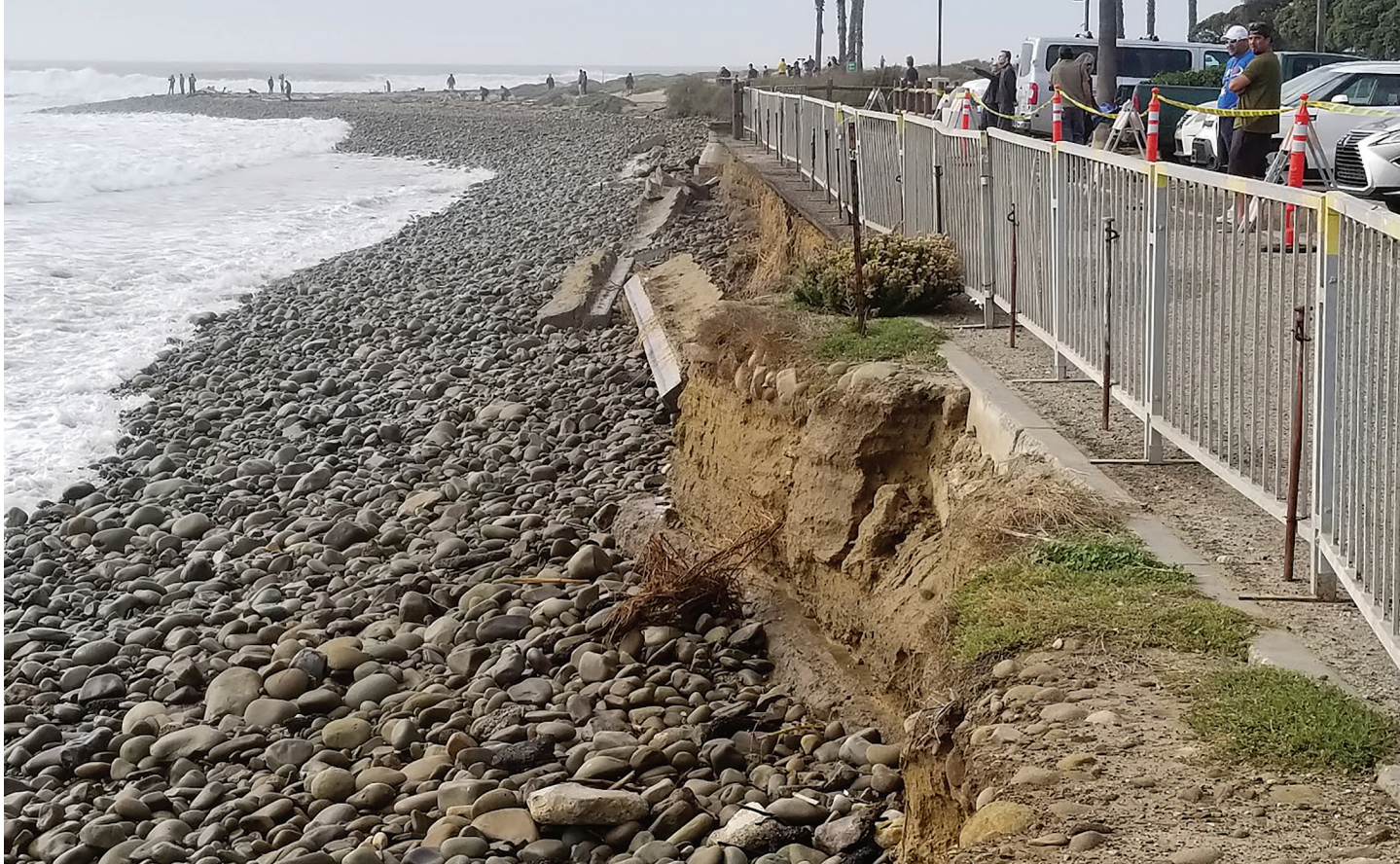
FIGURE 5. Erosion in Ventura, CA, threatens public access, parking, and public safety; a managed retreat project relying on nature-based solutions will increase access and parking.
