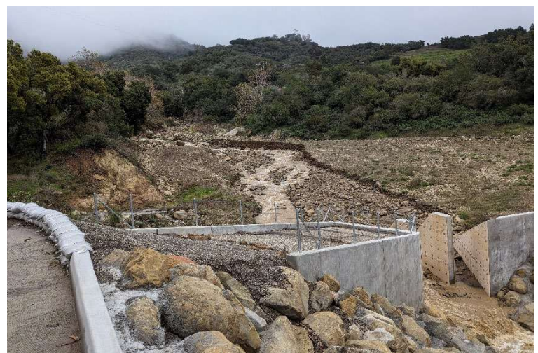
Figure 5-14. Romero Debris Basin, February 2024
