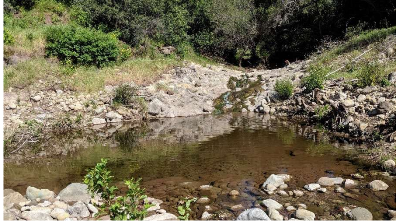
Figure 5-8. Original Main Branch Maria Ygnacio Debris Basin Inlet Grouted Rock Check Structure, looking upstream (April 10, 2019)
