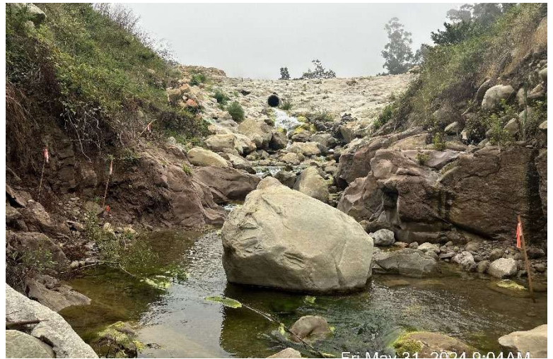
Figure 5-1. Original Cold Springs Debris Basin Embankment, looking upstream (May 2024)
