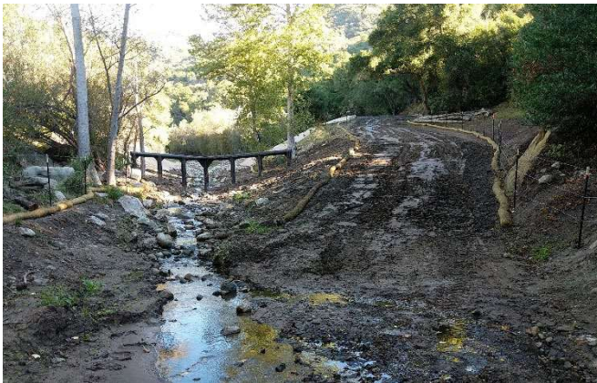
Figure 5-10. Modified Main Branch Maria Ygnacio Debris Basin, looking upstream (Dec 13, 2019)
