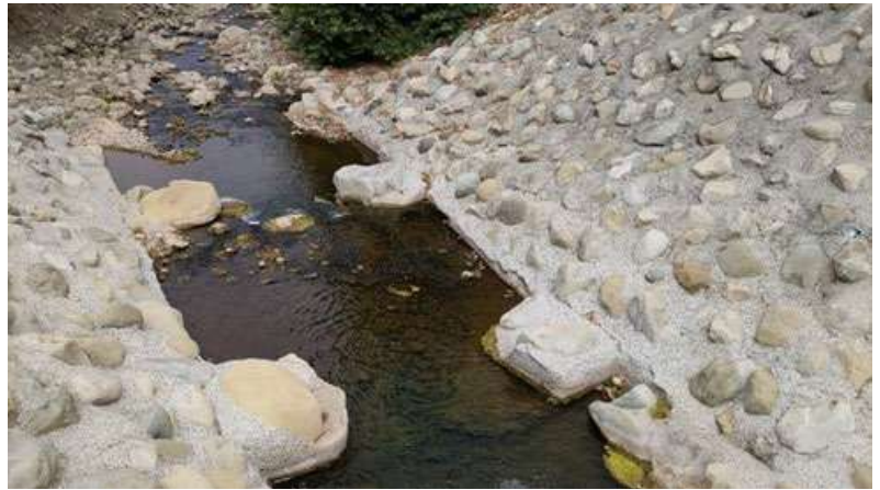
Figure 5-5. Modified Gobernador Debris Basin, looking downstream (Aug 2024)
