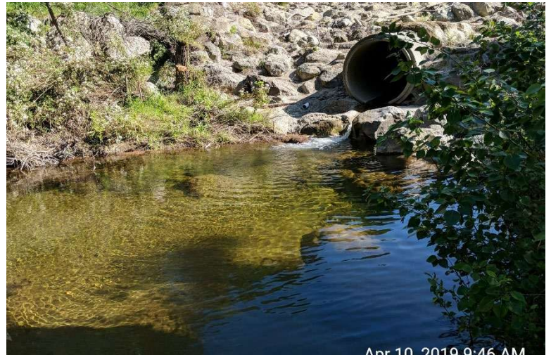
Figure 5-9. Original Main Branch Maria Ygnacio Basin Embankment, looking upstream (April 10, 2019)
