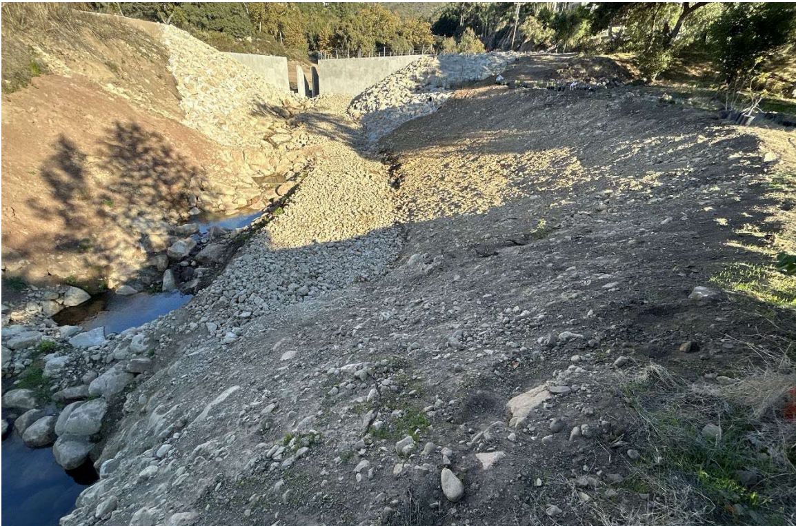
Figure 3-1. Hard structures (retaining walls, debris walls, grouted rock)
