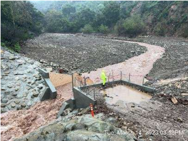
Figure 5-7. Post-Modification Gobernador Debris Basin, looking into basin (March 2023)
