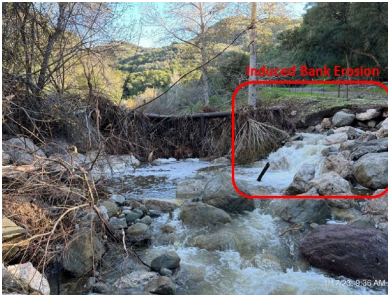
Figure 2-7. Debris rack in operation.
