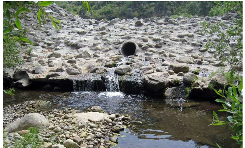
Figure 5-6. Original Gobernador Debris Basin Embankment, looking upstream (May 2008)
