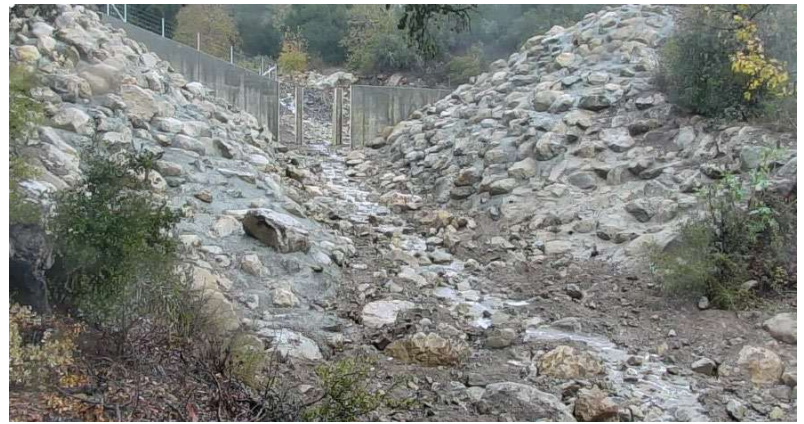
Figure 5-13. Post-Modification Romero Debris Basin, looking upstream
