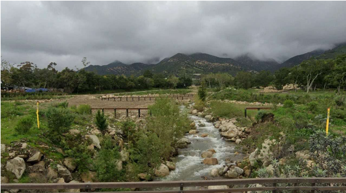
Figure 3-2. Minimal hard structures (open outlet with debris racks).
