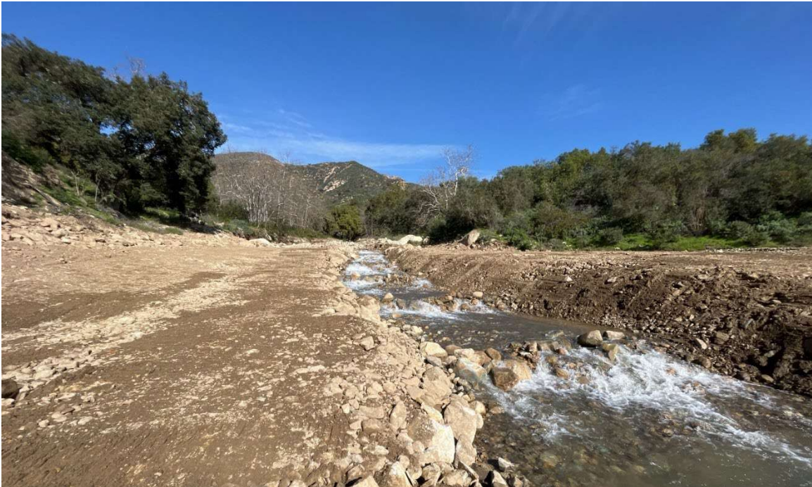
Figure 2-3. Basin pilot channel.
