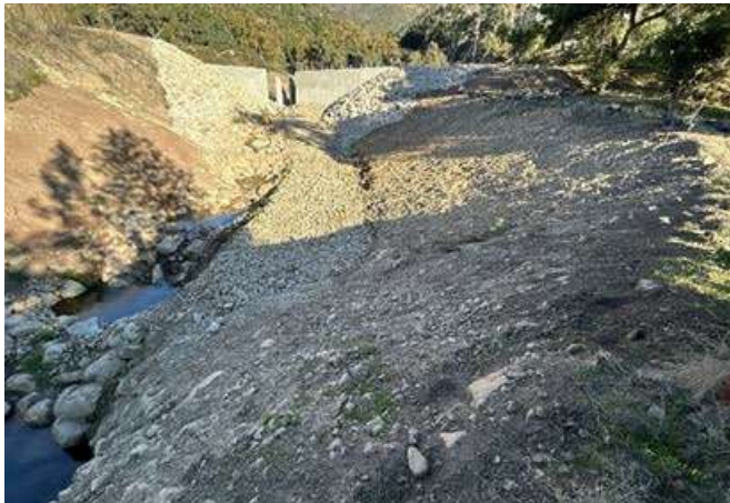
Figure 5-3. Post-Modification Cold Springs Debris Basin Downstream Improvements, looking upstream (Dec 2024)
