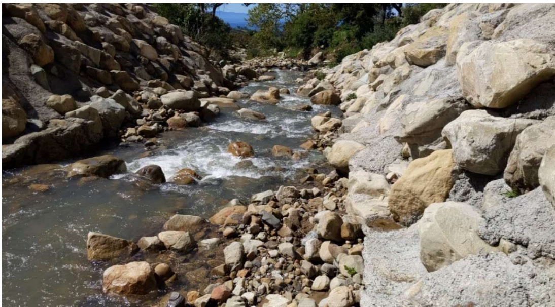
Figure 3-8. Rock ramp / roughened channel.
