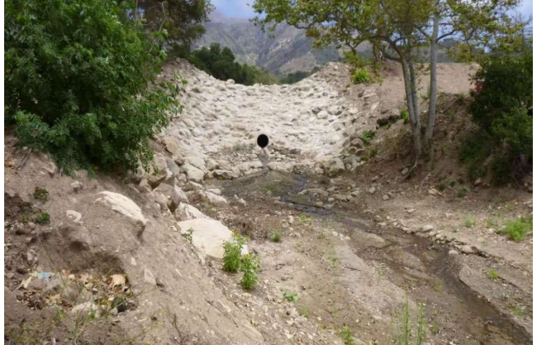
Figure 5-12. Original Romero Debris Basin Embankment, looking upstream
