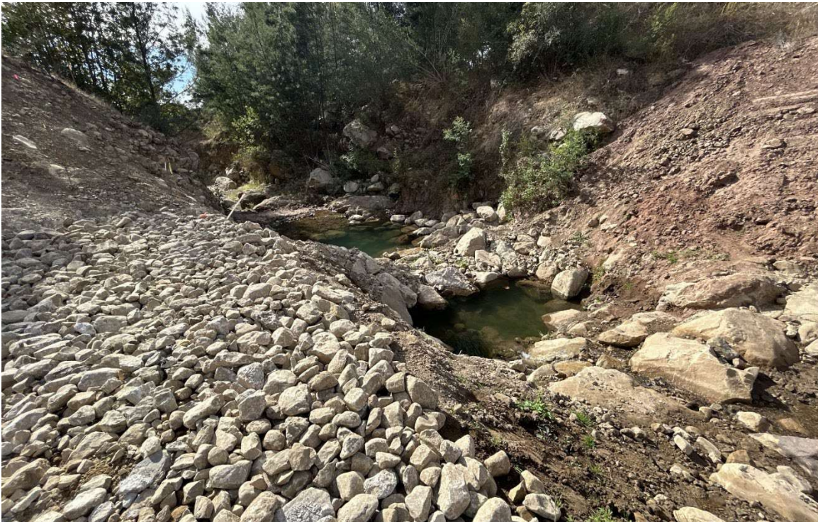
Figure 3-9. Step-pool/chute and pool channel.
