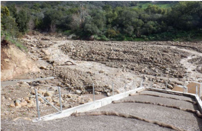
Figure 5-15. Romero Debris Basin during Jan. 2023 flood event
