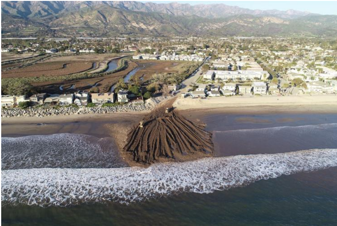
Figure 28 Image of sediment debris flow placement at the end of Ash Avenue in Carpinteria
