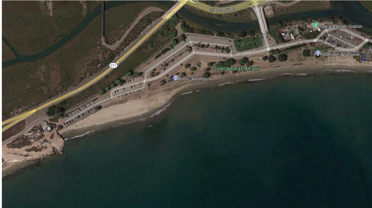
Figure 26 Aerial image of Goleta Beach on 8/19/2019 showing effectiveness of cobble groin at retaining sand.
