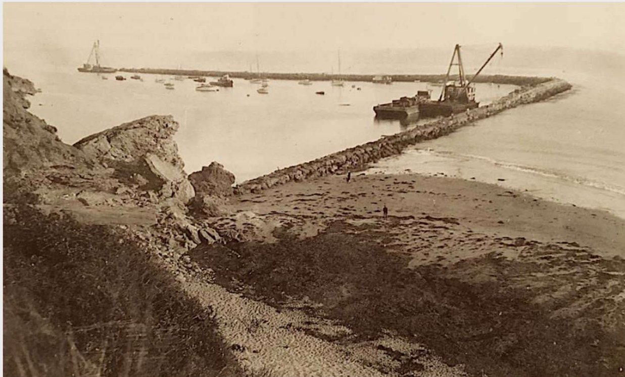
Building of the Breakwater
