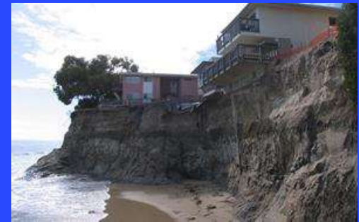
Eroding bluffs in Santa Barbara
