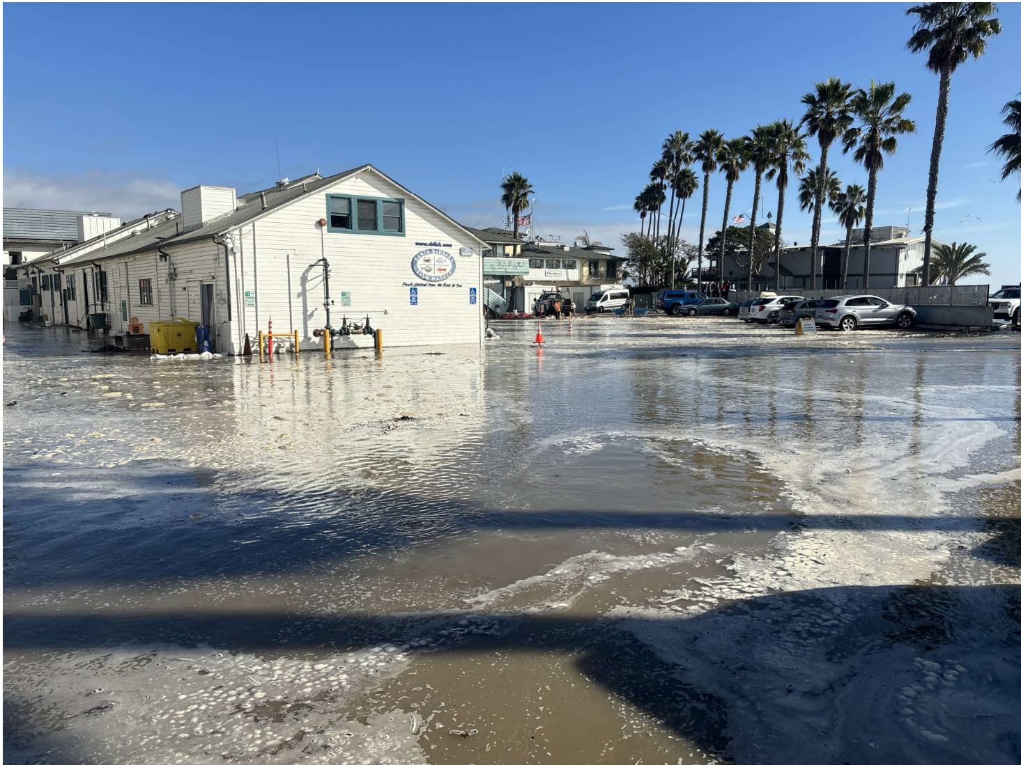
Harbor Business Area Flooded During High Tide & Swell
