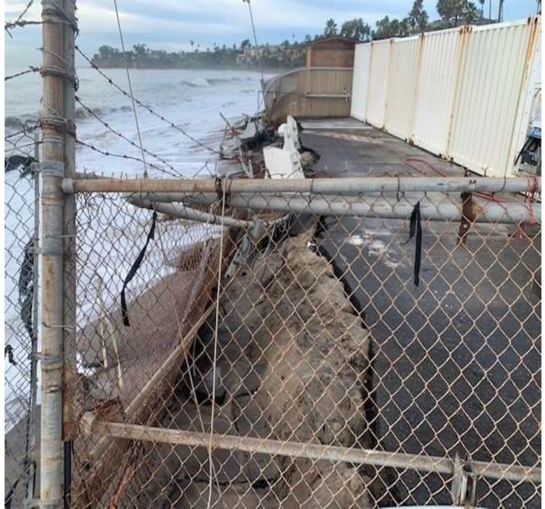
Coastal Infrastructure Damage Due to High Tide and Swell
