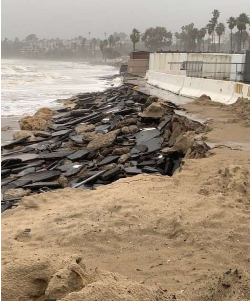
Coastal Infrastructure Damage Due to High Tide and Swell
