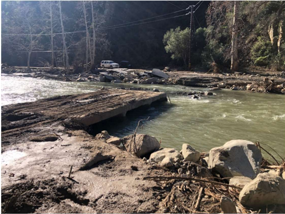
Camino Cielo Bridge – Ventura River (VCPWA-WP photo)
