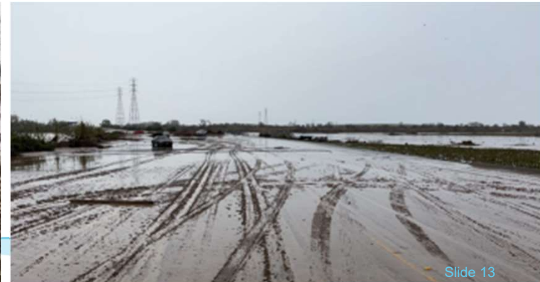
Victoria Ave Flooding (VCPWA-WP)
