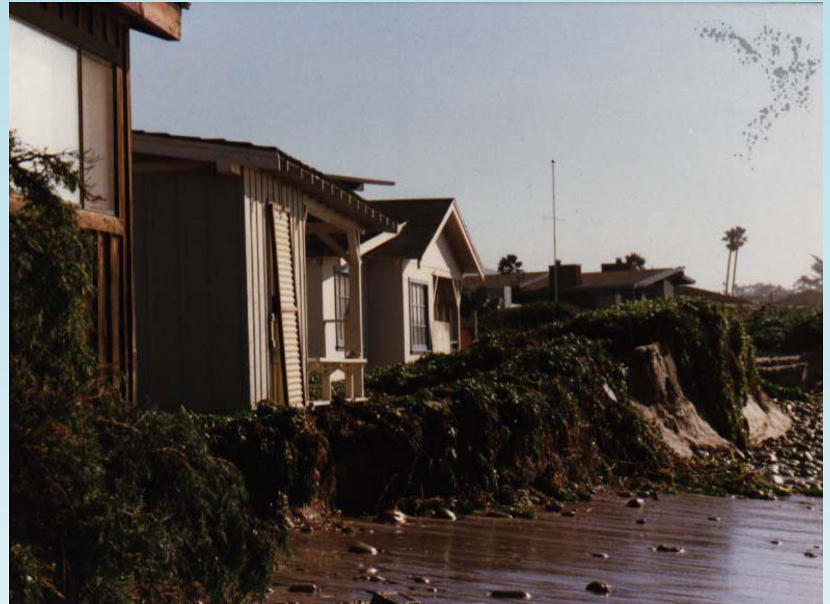
Coastal erosion and damage during historically large El Niño of 1982-83.
