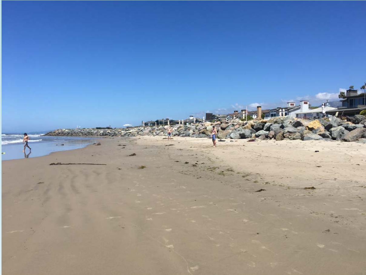
Rock revetment upcoast on County property
