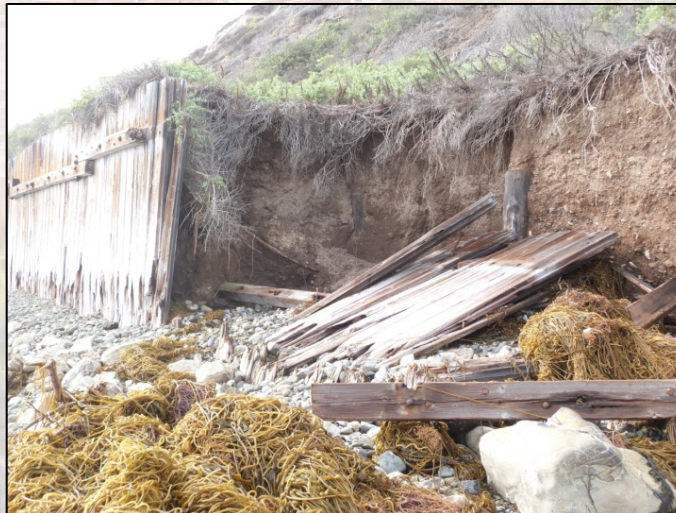
Broken and Eroding Old Oil and Gas Sea Walls on Ellwood Beach
