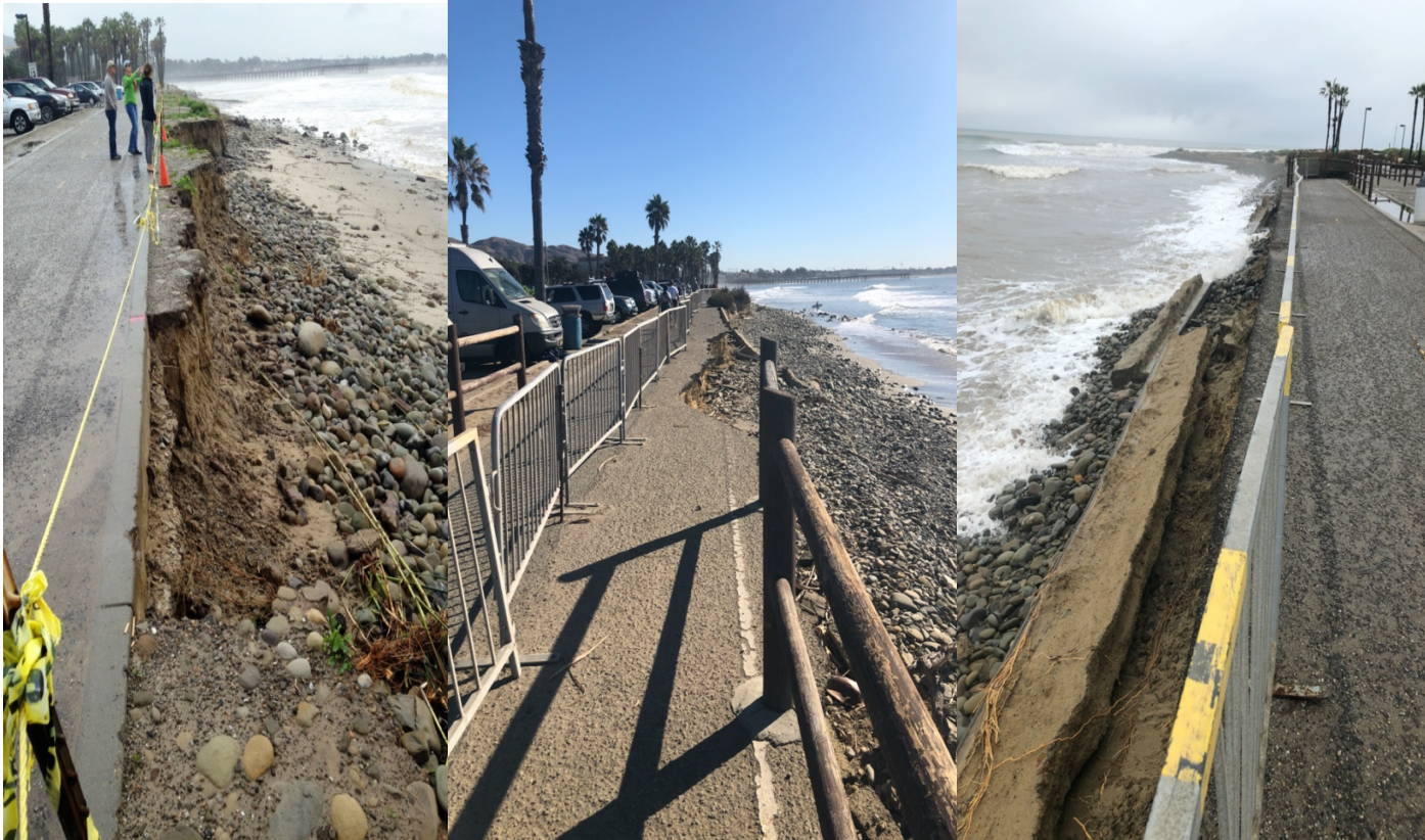
Phase 2 Surfer's Point Project Area: Continued Beach Erosion and Bike path damage from 2017-2019
